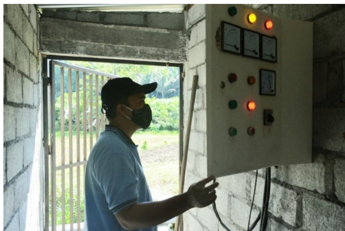
Figure 4. Installation of Solar Panels on Irrigation Systems
